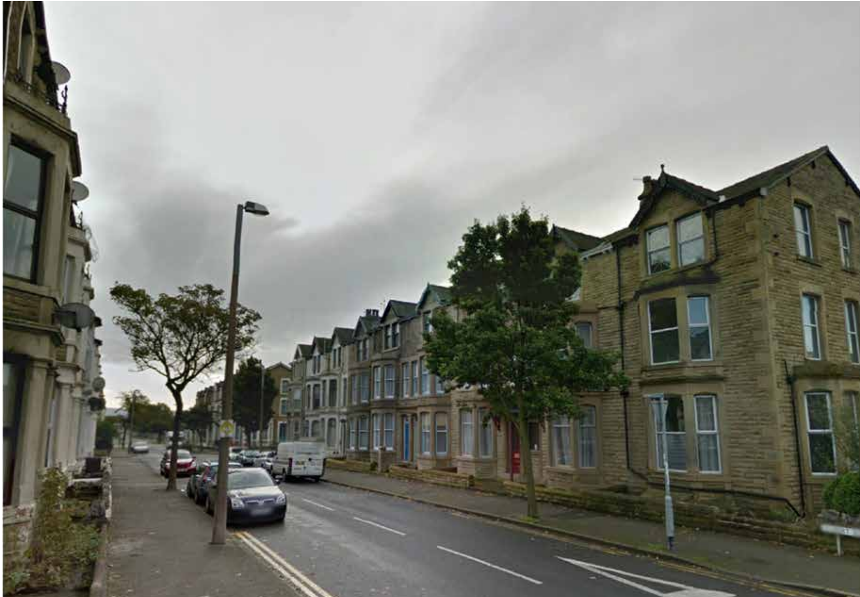
FIG.6 ALBERT ROAD (EXISTING) | TIRED PUBLIC REALM
